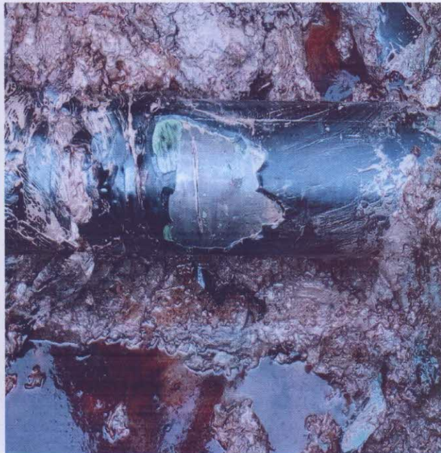
Fig B: Incident Facility after excavation
