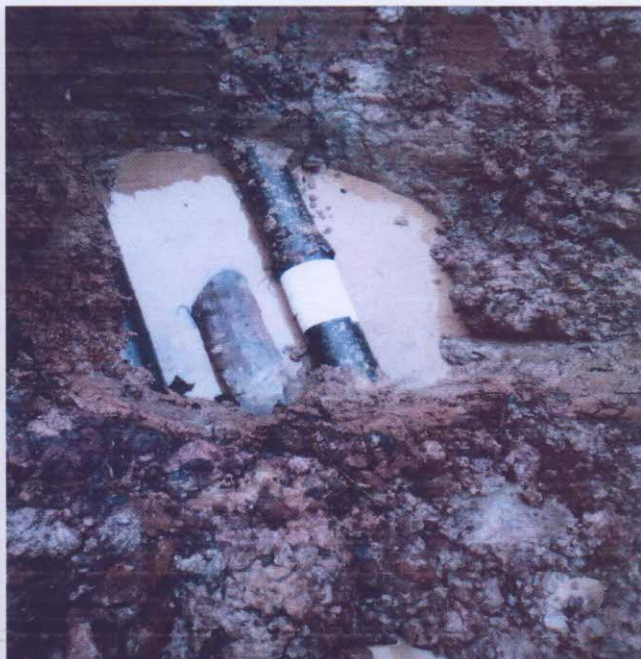
Fig D: Incident facility shortly after repair
